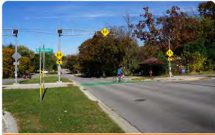
While cars may only turn right onto Whitney Way, shared-use path users can use the RRFB signal to safely cross the street to continue down Hammersley Rd.
