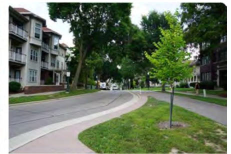
Road diets at Wilson and Broom made room for two bi-directional cycle tracks, accompanied by sidewalks.
