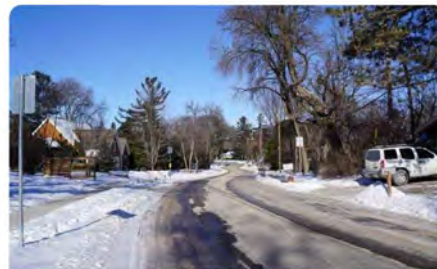
Winding streets slow drivers down. This stretch of Lake Mendota Drive used to be a straightaway—to prevent speeding, the City installed bump outs and added slight turns.
