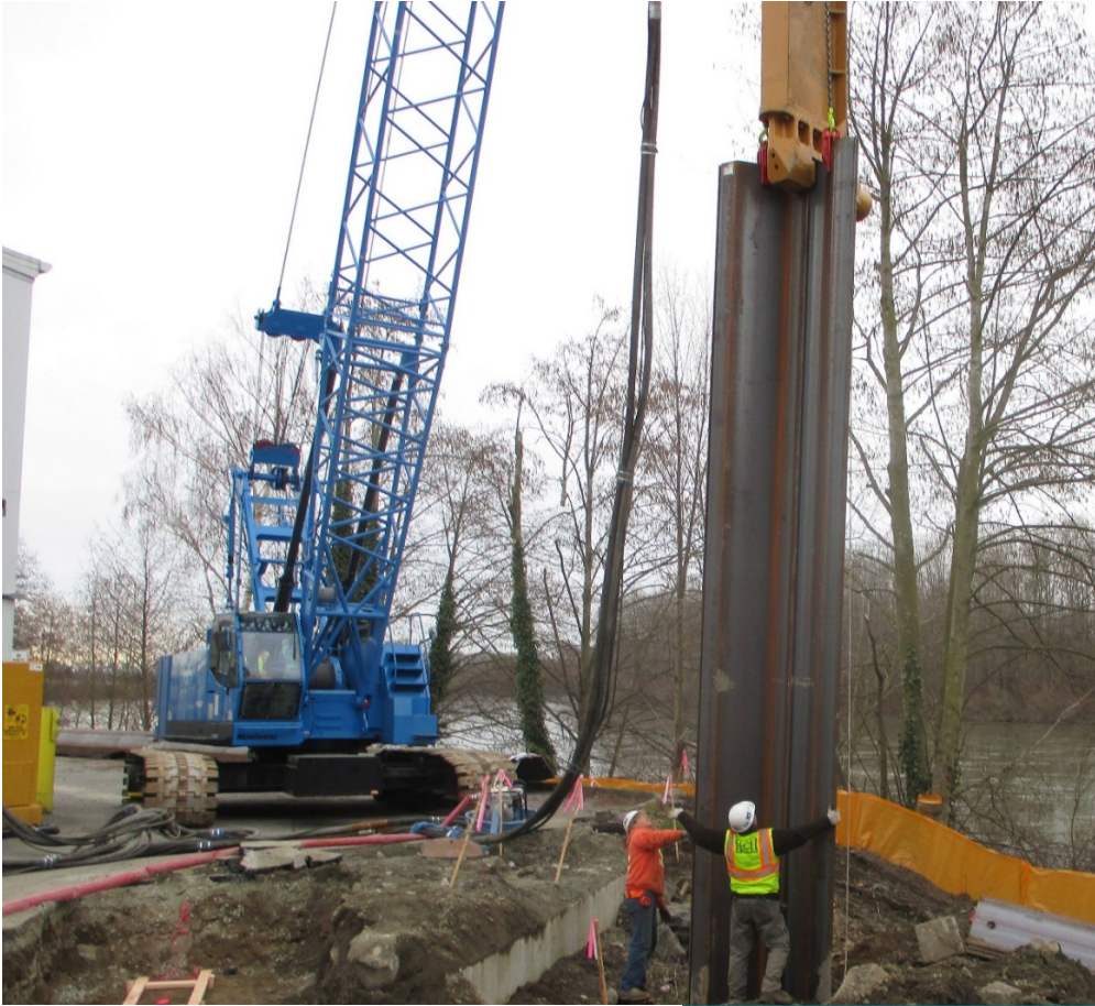
Top: Crews installing the Sheet piling.
