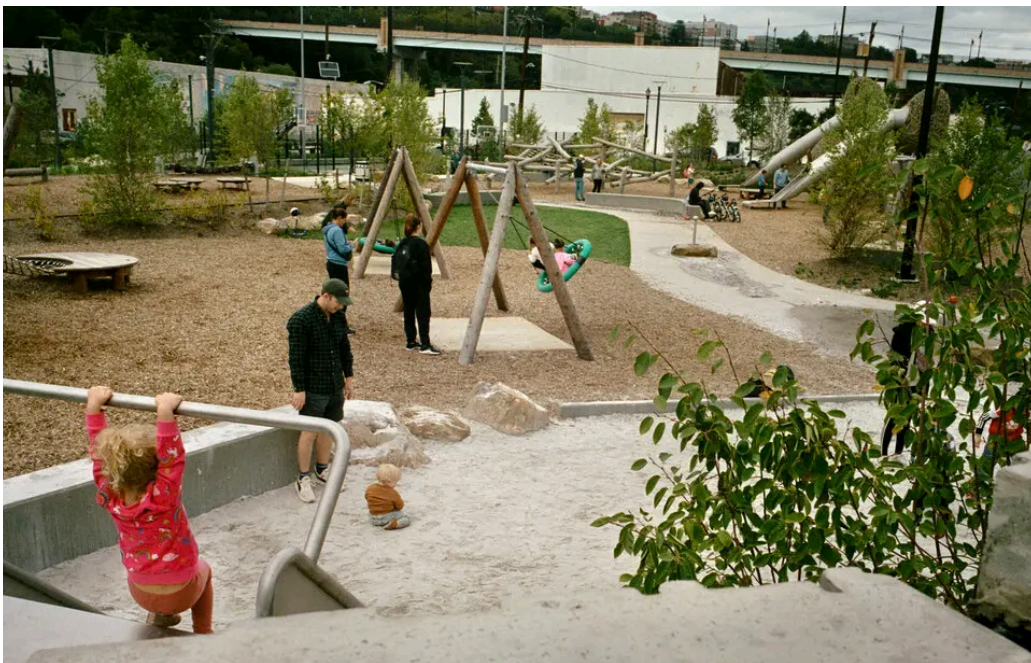
The new ResilienCity Park has playgrounds and fields — and the storage tanks underneath collected 1.4 million gallons of water during the September storm.
