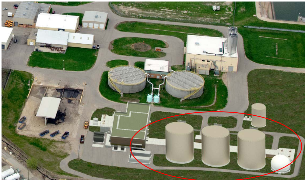
WRRF biodigester groundbreaking
