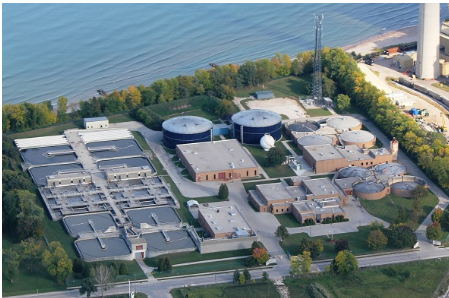
Sheboygan Regional Wastewater Treatment Facility; http://www.sheboyganwwtp.com/
