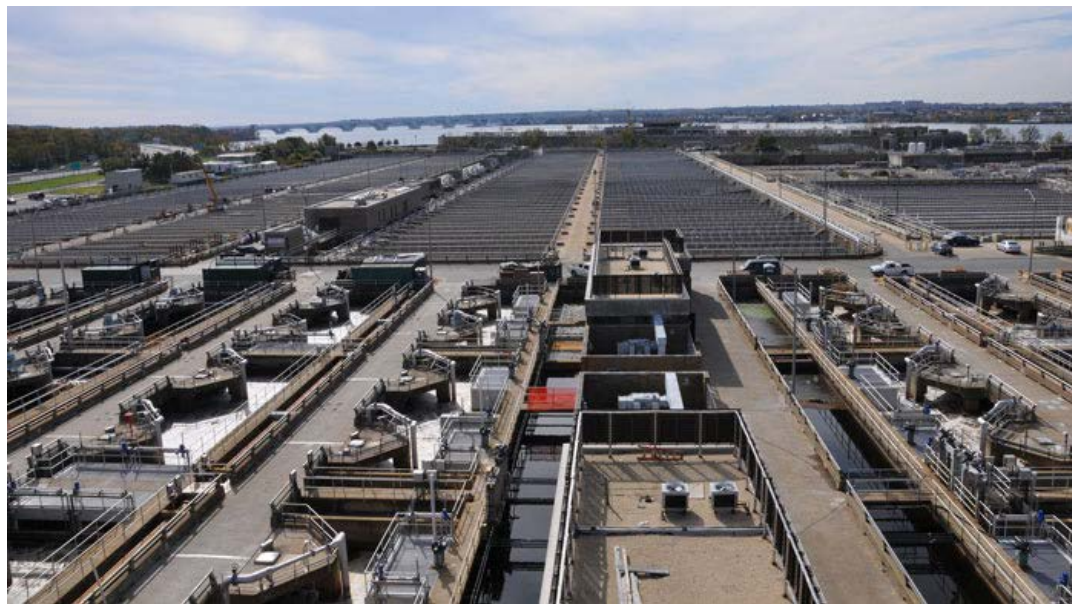
Blue Plains wastewater treatment plant, Washington, DC
